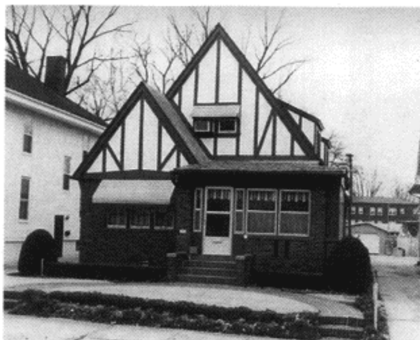
Built: 1927 Architecture: Tudor Revival
