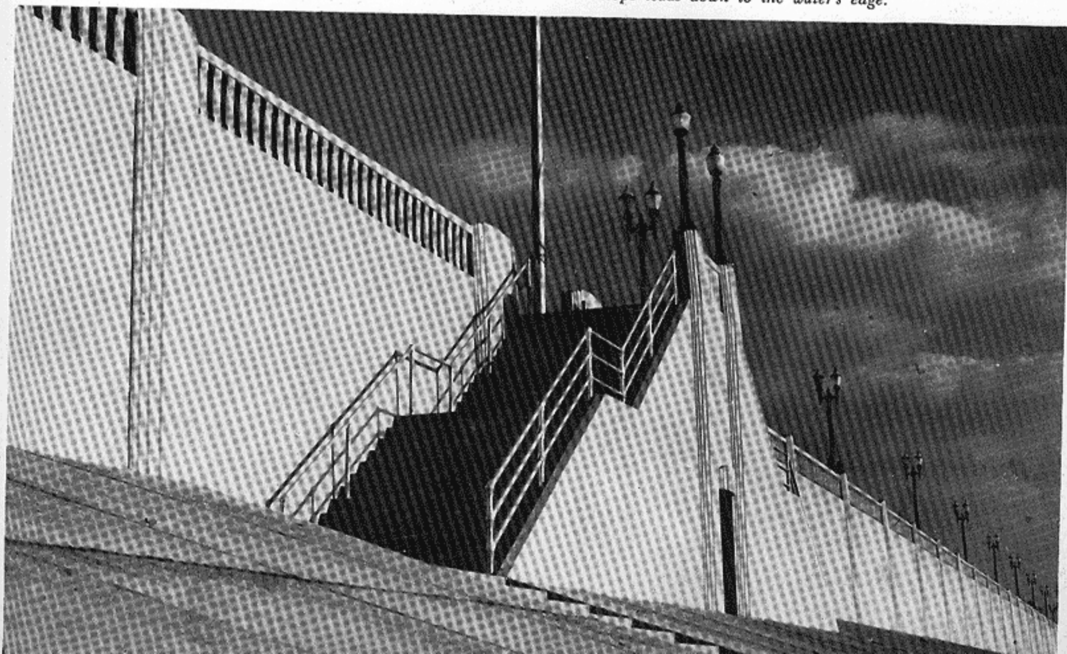
Dress Plaza extends along Evansville's "front yard" which overlooks a sweeping crescent curve in the Ohio River. An auto drive on the concrete slope leads down to the water's edge.
