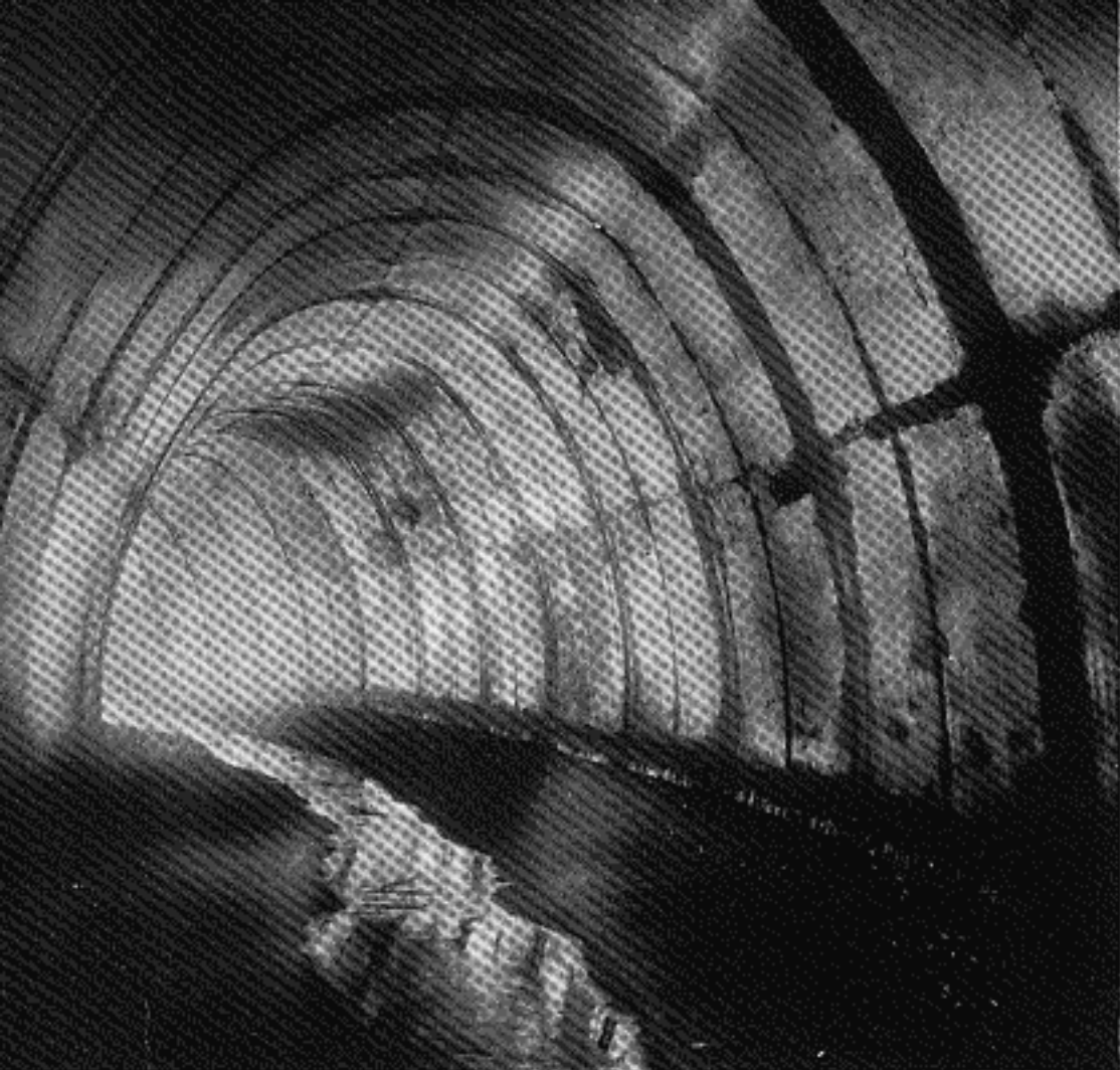
Holland-Tunnel-like is this Evansville sewer, part of the city's excellent sanitation system.
