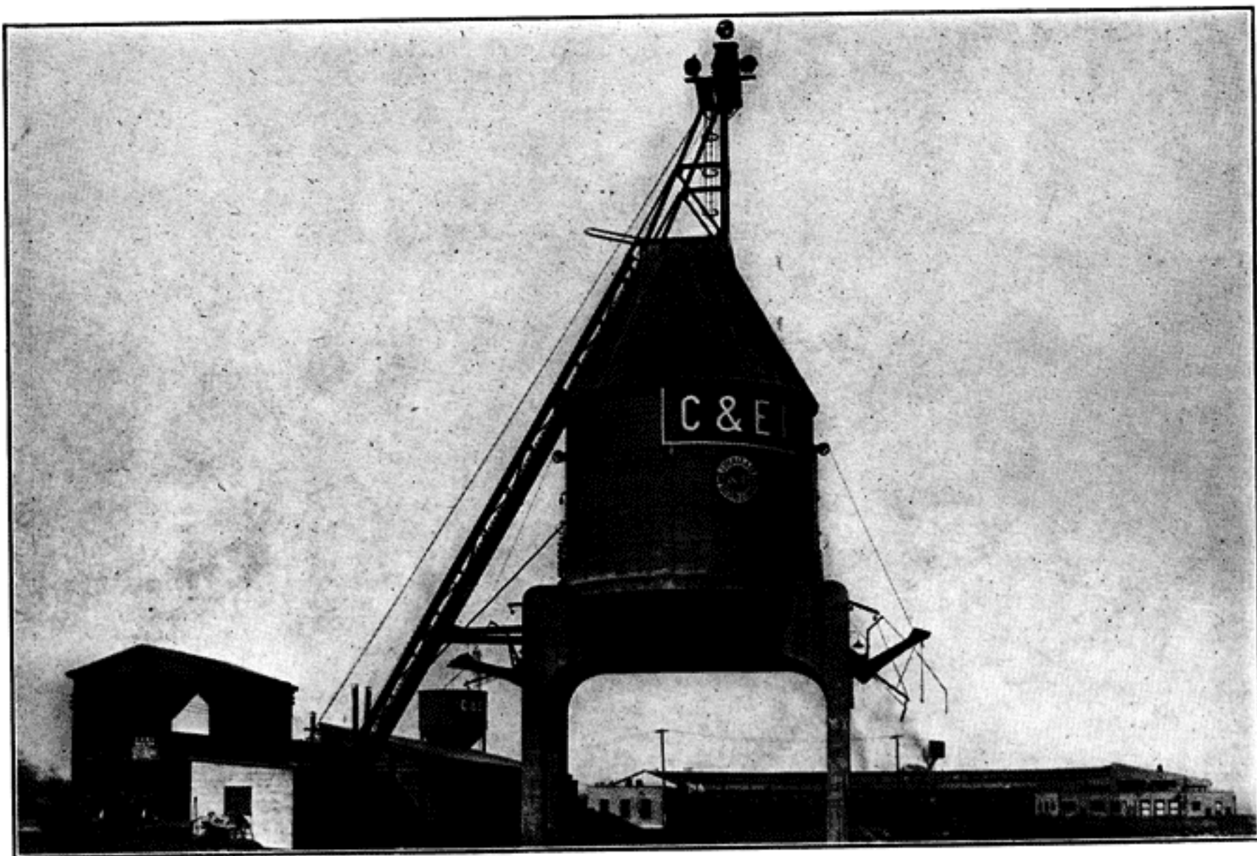
Engine handling facilities at new C. & E. I. Yard north of Pigeon Creek, showing modern coal chute in foreground, roundhouse in background.
