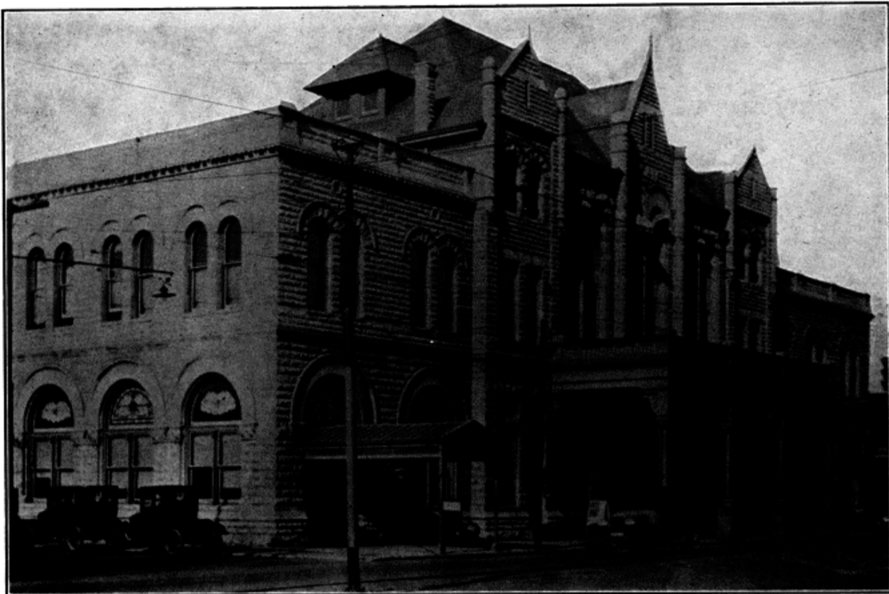
L. & N. Railroad Passenger Station; a suitable and conveniently arranged building. A station plaza opposite would be of immense benefit to the city.
