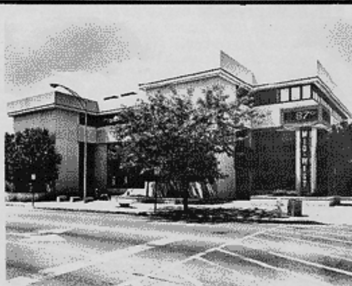
New Midwest Federal Building in the Riverside Project.
