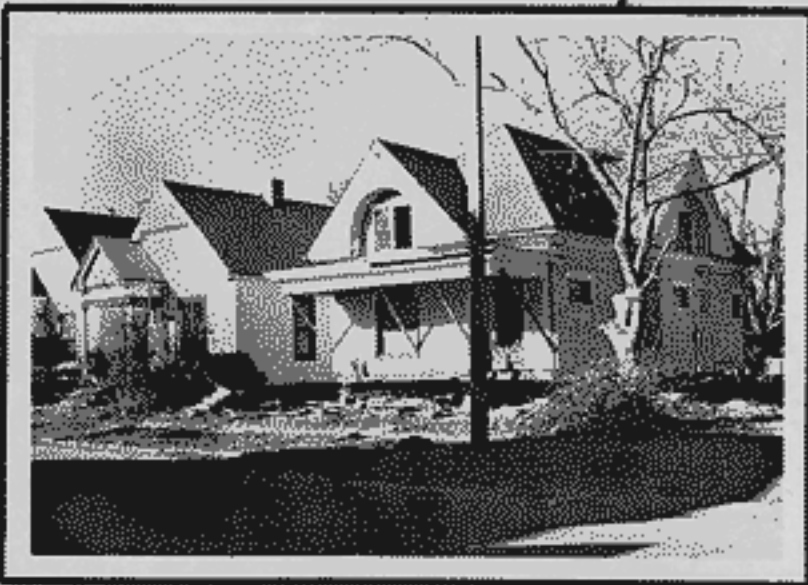
Goosetown Neighborhood house being moved to a vacant lot for rehabilitation and to make room for a mini-park.
