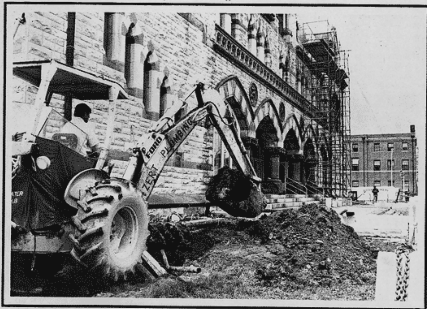
Work underway in $1,200,000 renovation of the Old Post Office.
