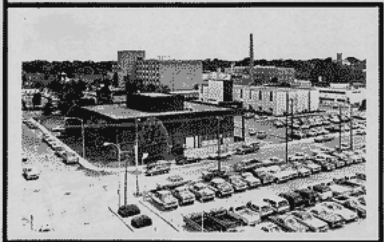
IBM Building (foreground), Welborn Clinic (right), and Welborn Baptist Hospital.
