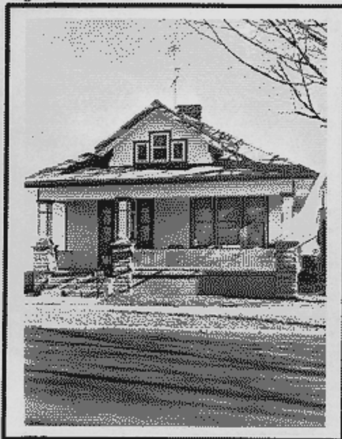
Completed rehabilitation in the Lincoln-Walnut Neighborhood.
