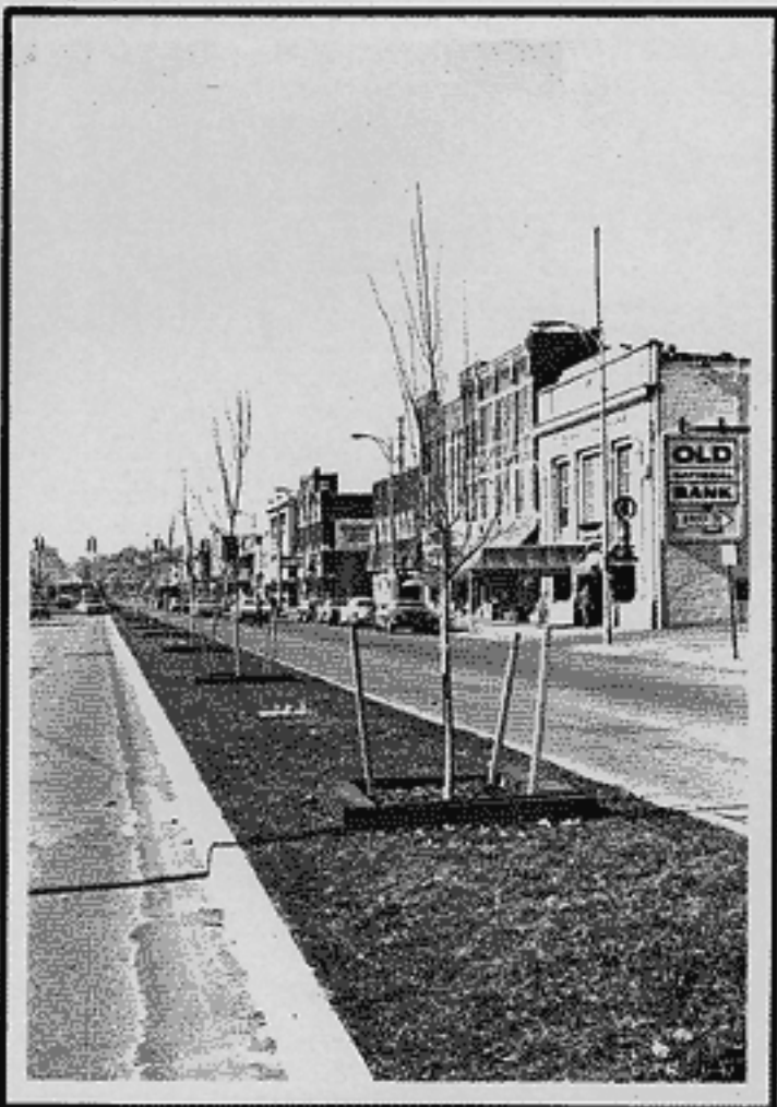
West Franklin median. Phase I of a commercial revitalization project.
