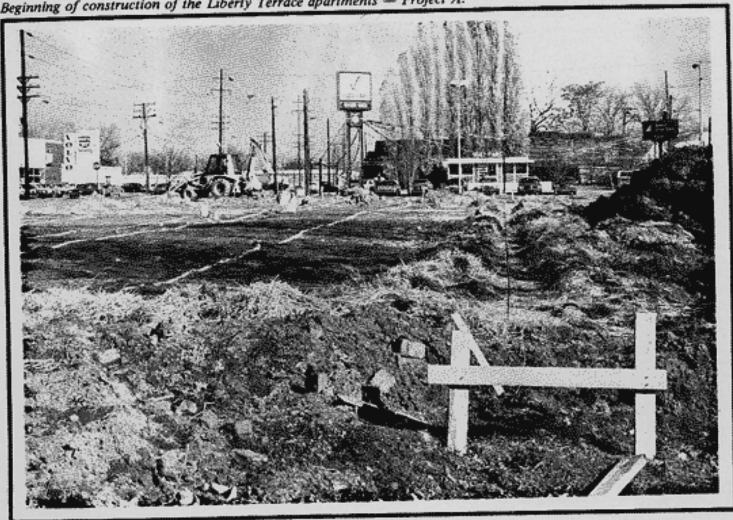
Beginning of construction of the Liberty Terrace apartments — Project A.
