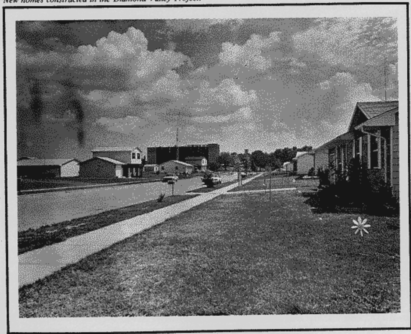
New homes constructed in the Diamond Valley Project.
