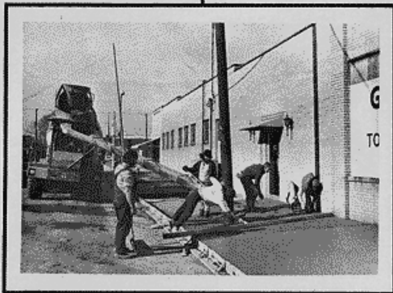
North Main public improvements. Phase I of a commercial revitalization project.
