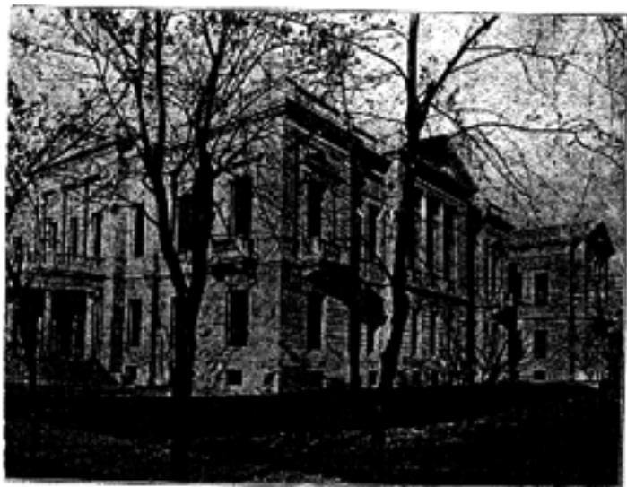
PENNSYLVANIA STATE LIBRARY AT HARRISBURG, PA. ERECTED OF GREEN RIVER STONE FROM CADEN STONE CO.'S QUARRIES.
