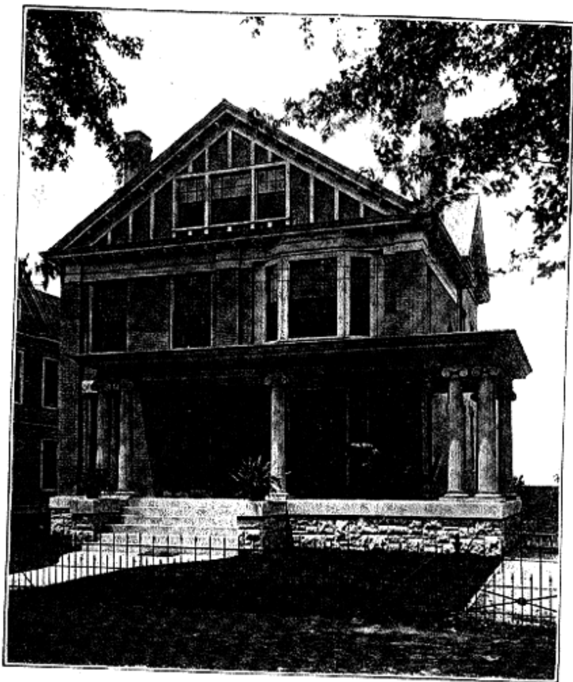
RESIDENCE A. B. JARVIS, HENDERSON, KY.
