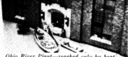
Ohio River Plant—reached only by boat
