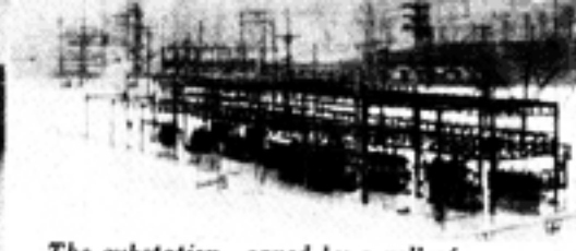
The substation—saved by a roll of canvas
