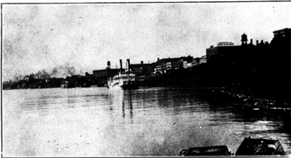
The need of a marginal wall and promenade along the river is clearly shown here.
