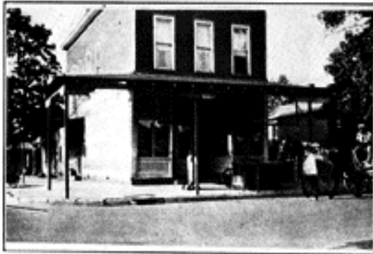
Sidewalk canopies such as this injure the city's appearance.
