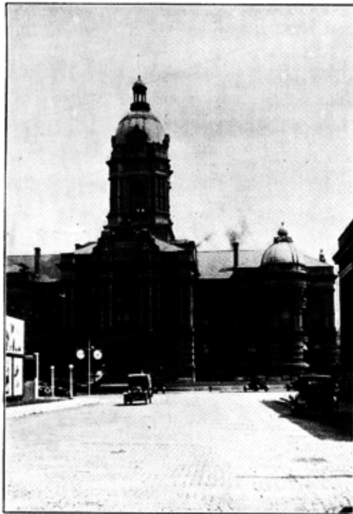
The Court house is a fine old building, injured by inadequate setting. It is almost impossible to find a place from which to see the whole building at once.
