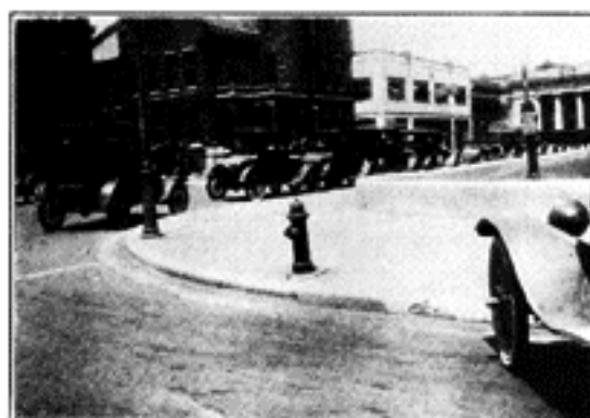
A well-rounded corner like this helps traffic and is pleasing to the eye.
