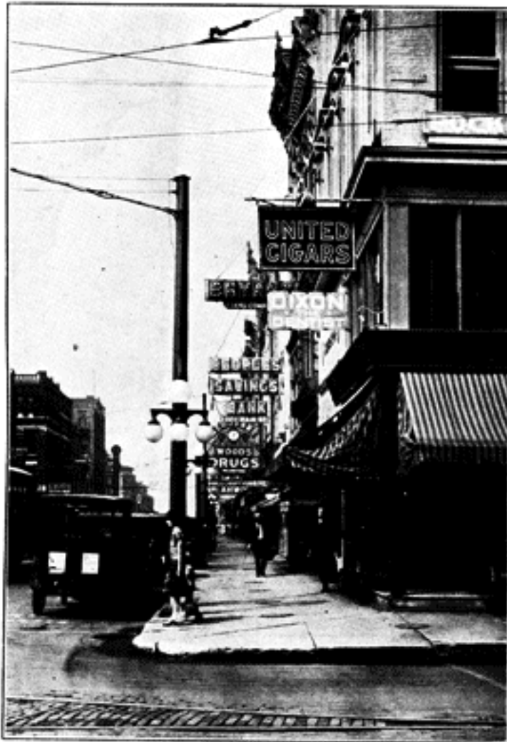
The use of many large overhanging signs is marring the appearance of the main business streets and at the same time reducing the effectiveness of this form of advertising.
