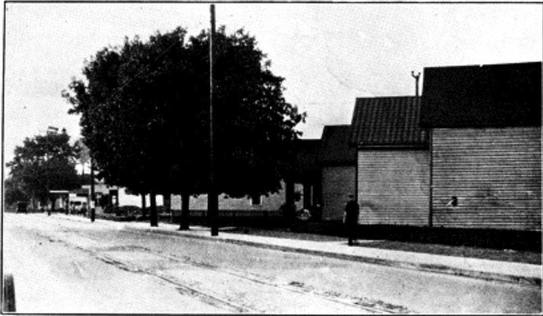
This saw-tooth arrangement of houses, due to poor land subdivision, spoils the appearance of the street and reduces the usefulness of the lots.
