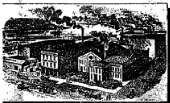
DESTROYED BY FIRE OCTOBER 16, 1891.
