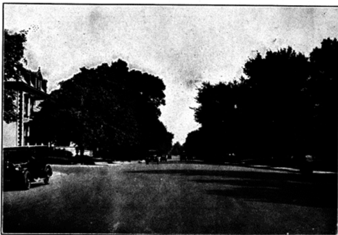
Riverside Avenue, illustrating the dignity and impressiveness of a wide boulevard. Note absence of poles and wires and the charm of tree masses.
