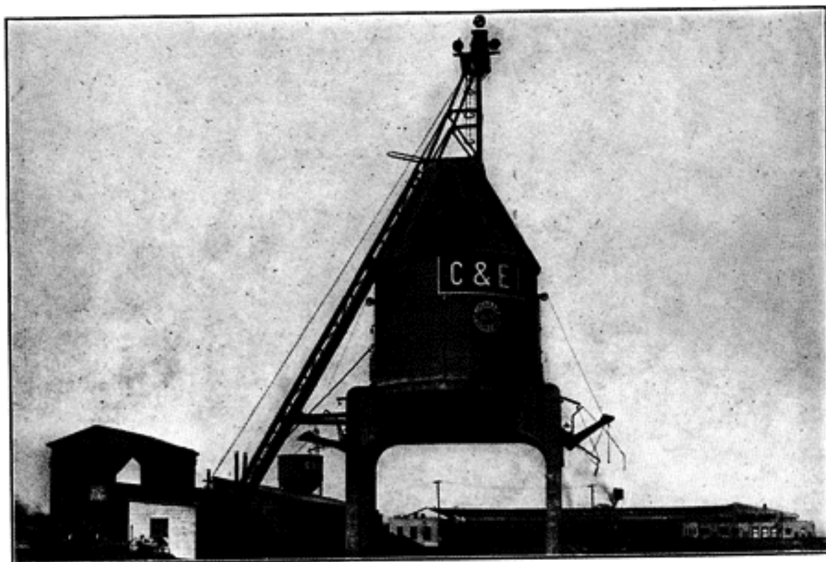
Engine handling facilities at new C. & E. I. Yard north of Pigeon Creek, showing modern coal chute in foreground, roundhouse in background.
